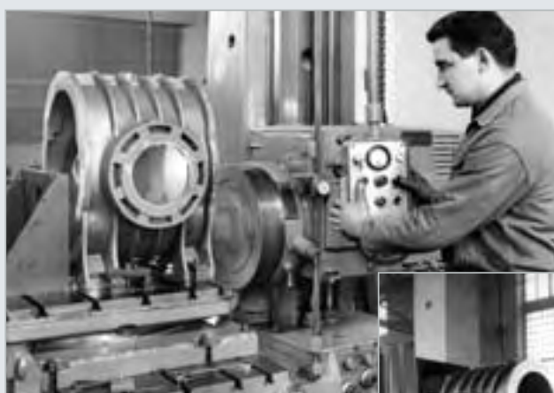
RORThe 60s: ROR blowers casing - sides manufacture
